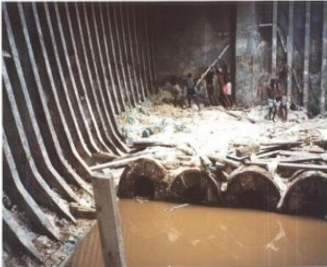
Figure 1: Cargo damage due to water ingress
